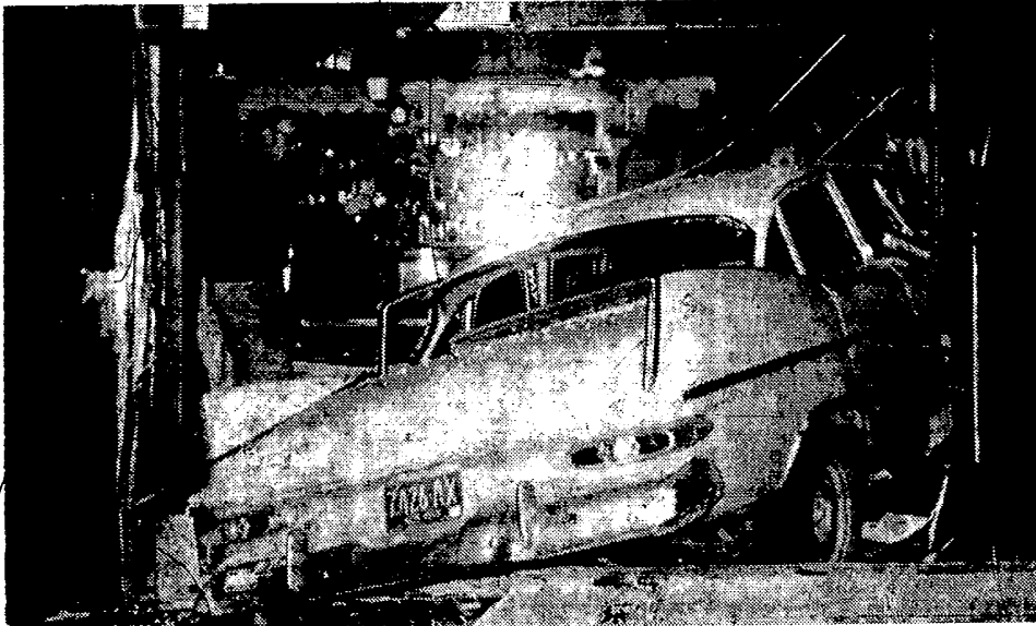
This view was taken from the "outside looking in" with a Gas Company Employee checking for gas leaks after the gas had been shut off. The license plate of the car, 7426 AX, identifies it as a car that came from Allegany County.
